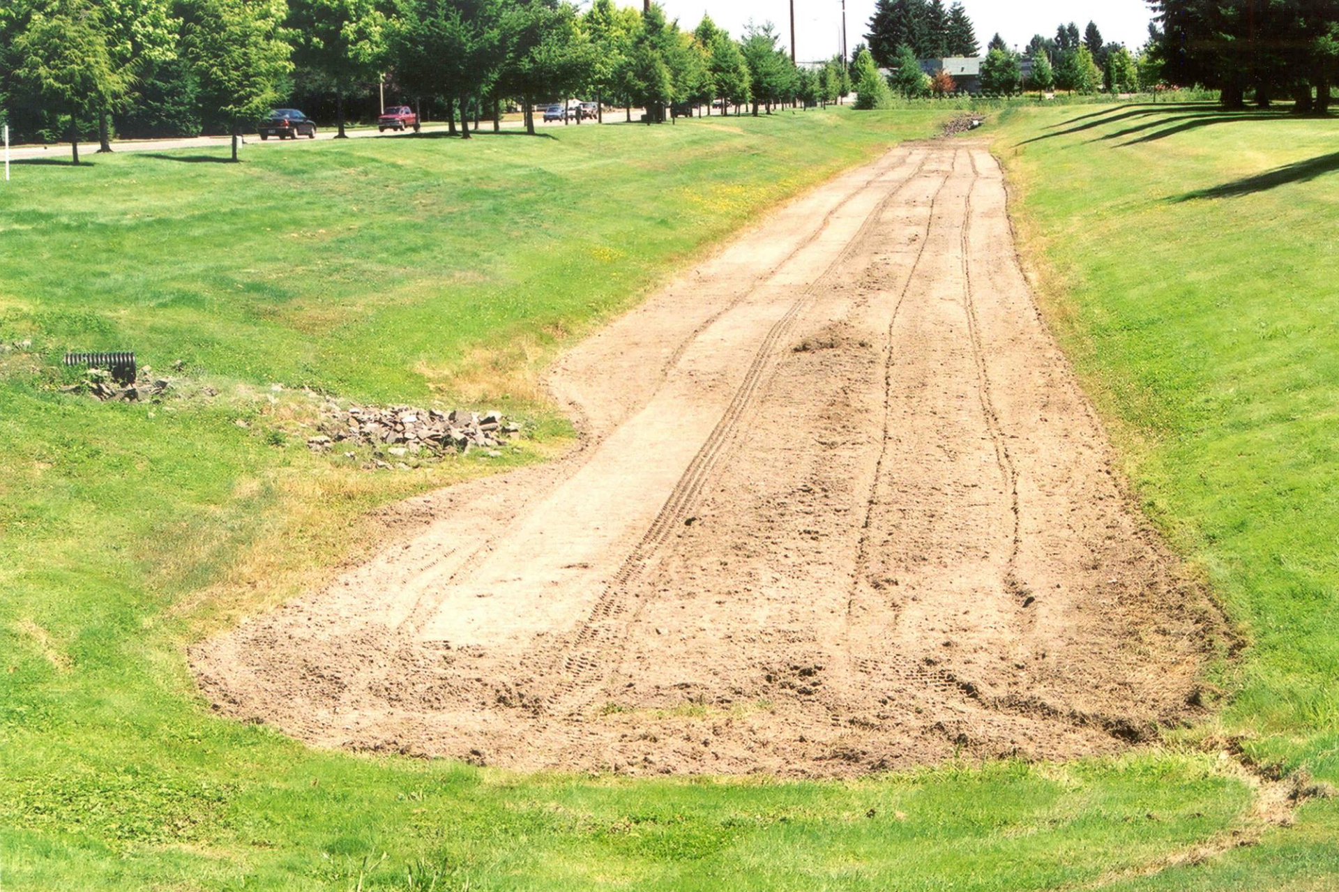
Biofiltration Swale During Construction
